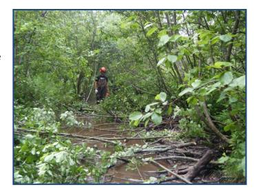
In general, the stream was about four times as wide and four times as shallow as it should have been. There were almost no holes or undercuts where fish could find cover in the upper regions. The work crew removed alders and blockages on about two-thirds of the river, not counting the ponds. This aspect of the project was very effective.
