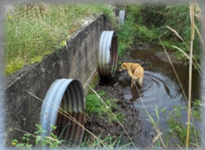
Picture: Winter River at Union Road Pumping station.
