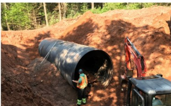
Work continues to restore fish passage
