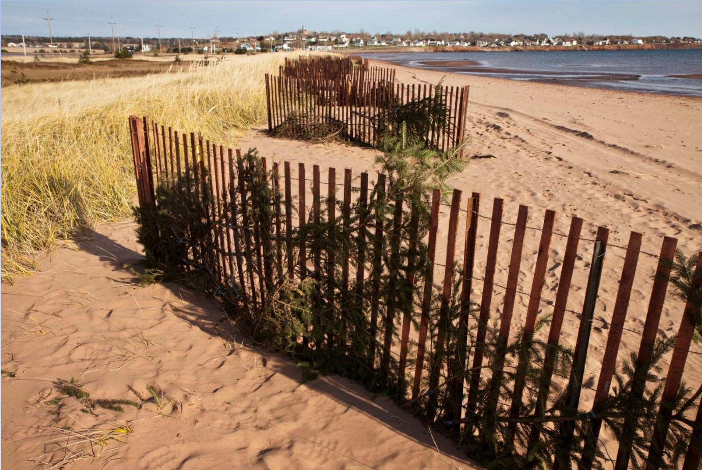
Souris Wildlife Federation sand nourishment method to build up sand on the Souris Causeway
