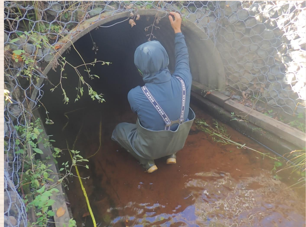
Evan checking inside of culvert.
